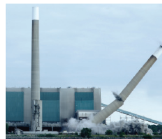
Figure 10.13 (Conceptual Example 10.5) A falling smokestack breaks at some point along its length.
