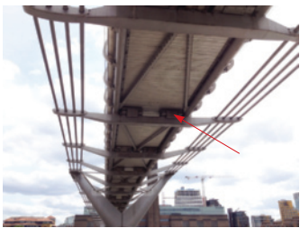
Figure 15.20 The London Millennium Bridge over the River Thames in London. On opening day of the bridge, pedestrians noticed a swinging motion of the bridge, leading to its being named the "Wobbly Bridge." The bridge was closed after two days and remained closed for two years. Over 50 tuned mass dampers were added to the bridge: the pairs of spring-loaded structures on top of the cross members (arrow).
